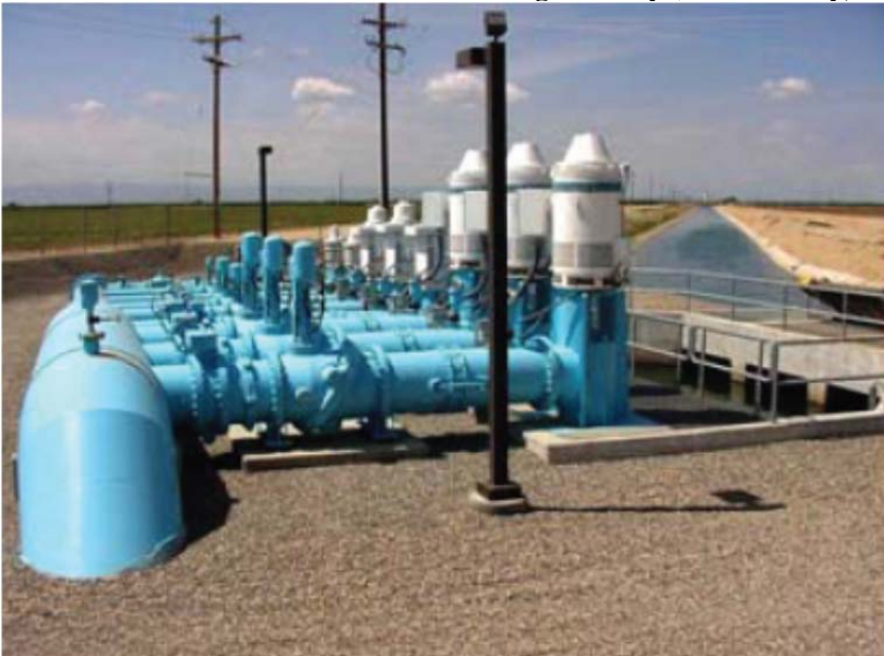
FIGURE 3 – In-Lieu Groundwater Recharge Facility (Kern County, California)
